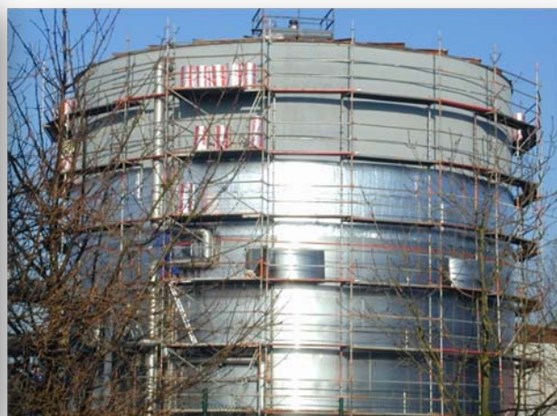
The whole tank was insulated after the application.
