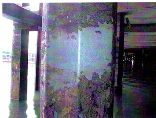
Plate 1. Area of pile cleaned for inspection
